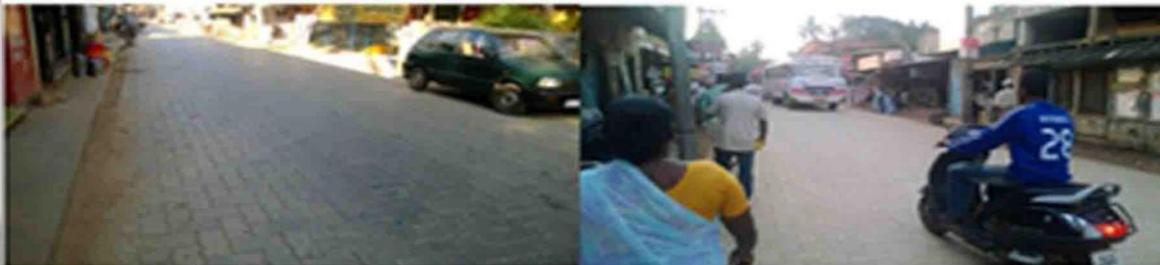
Fig.2. Condition after the construction using Interlocking concrete Blocks at Vakkom Market Jn.
