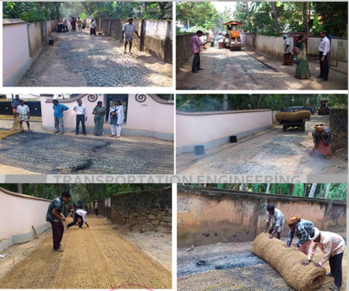
Field implementation of geotextiles
